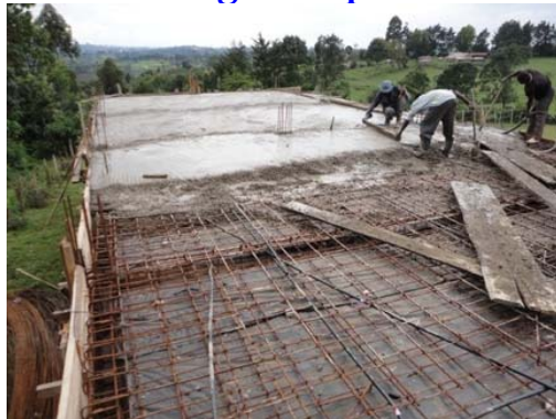
In the photo, the worker was finalizing the floor
