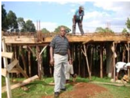
Remmy Koech standing by the construction site
